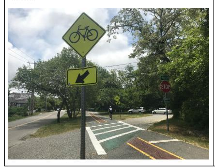
Figure 102: Image of Path Crossing the Southern Leg of the Y Intersection (Jones Road). Note the Bike Trail Crossing Signage and Ladder Crosswalk
